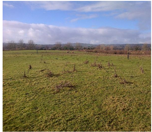
Landfill surface showing passive vent pipes
