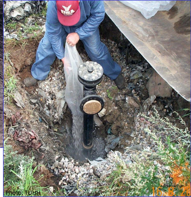
Installation of the clay cap
